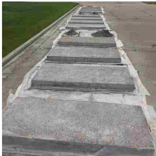
Figure 6-1 Concrete pavement sections as substrate
