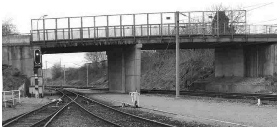
Figure 2-8 General view of the existing bridge (Matteis et al., 2008)
