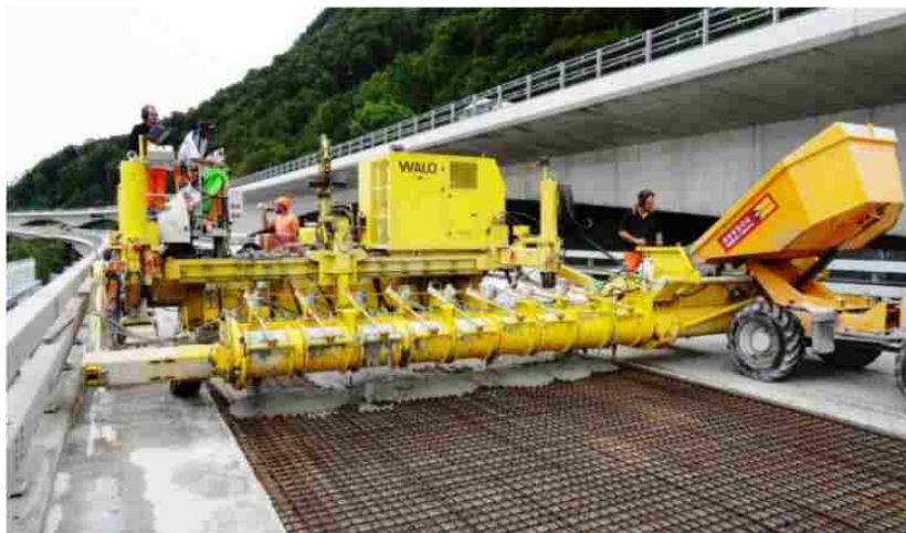
Figure 2-16 Implementation details of UHPC overlay application
