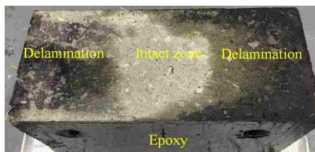
Figure 10- Photo of the overlay-substrate interface after the dye test
